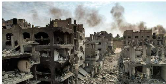
This picture taken on October 11 2023 shows an aerial view of buildings destroyed by Israeli air strikes in the Jabalia camp for Palestinian refugees in Gaza City. Yahya Hassouna / AFP via Getty Images
